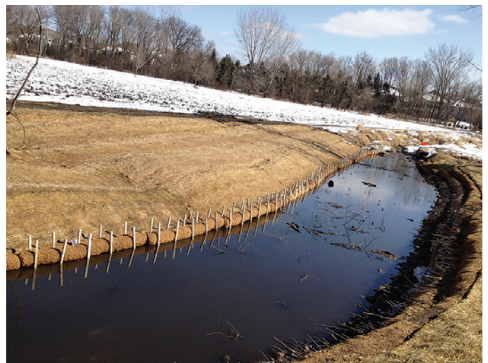
EG 2C-NN & Koir Log on a stream bank site
