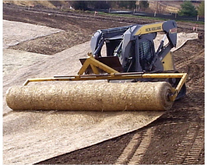
EG 2S - 1000 sy roll installation
